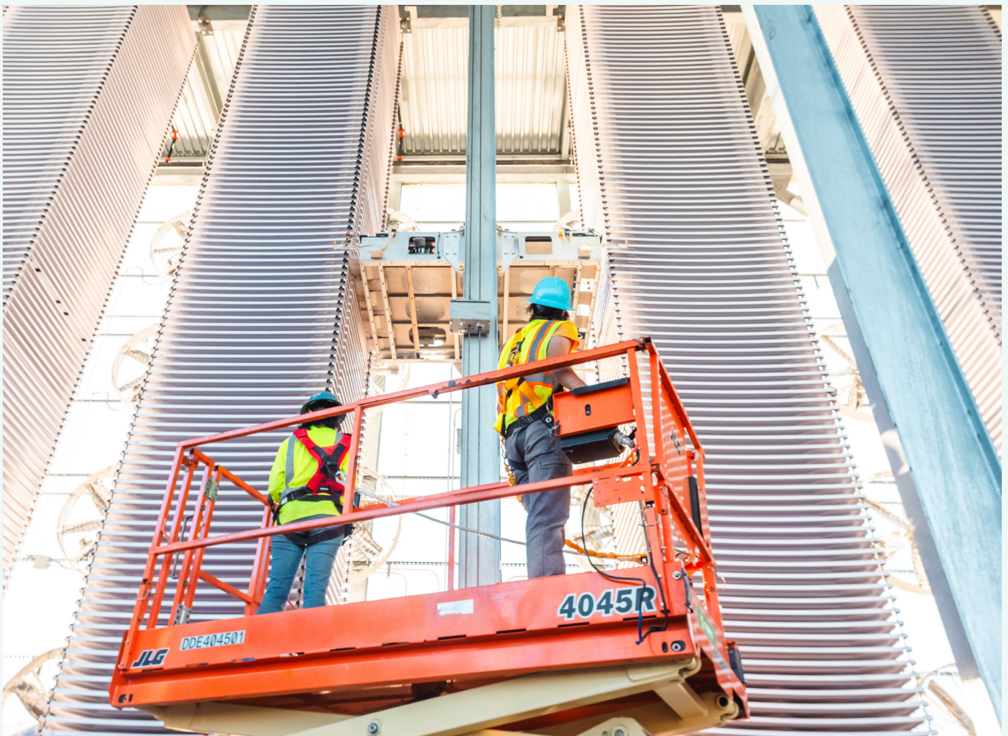
A safety team completes contactor inspections at Heirloom's Direct Air Capture facility
